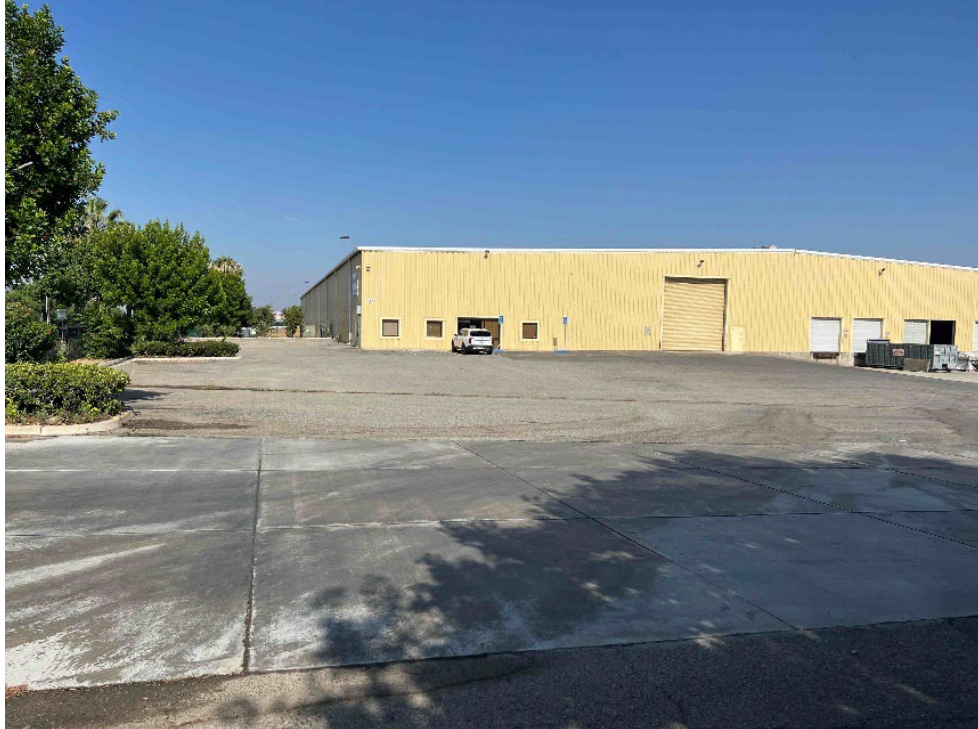
Photo 1: Overview of parking area and existing warehouse in the south-central portion of the project site, facing west.
