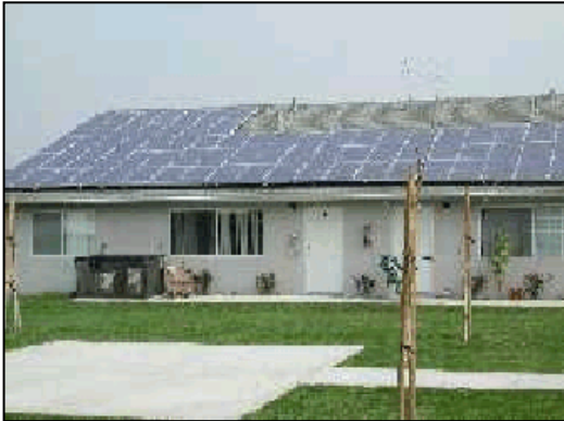
Rooftop solar panels provide clean electricity to homeowners.
