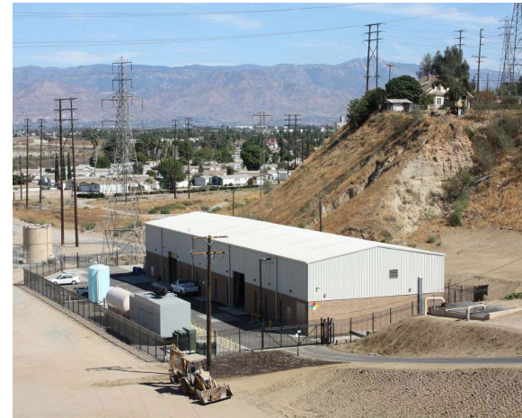
John North Water Treatment Plant
