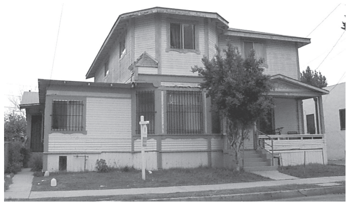
Inappropriate Addition to Front Facade
