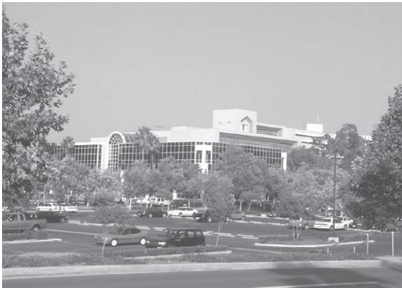
Riverside Community Hospital, 1990's wing
