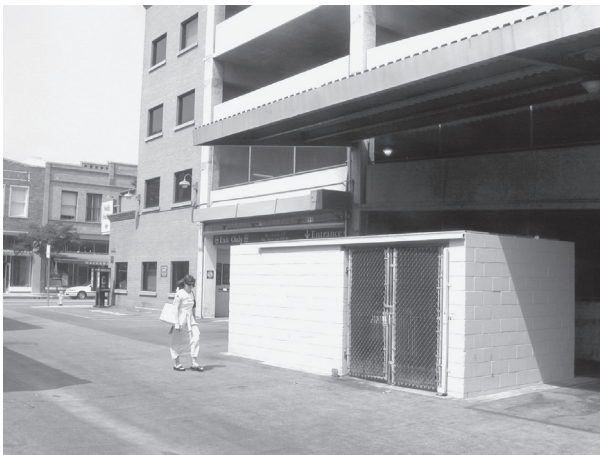
Alley walkways can also provide access to centralized trash compactors serving an entire block. These compactors are built into parking structures.
