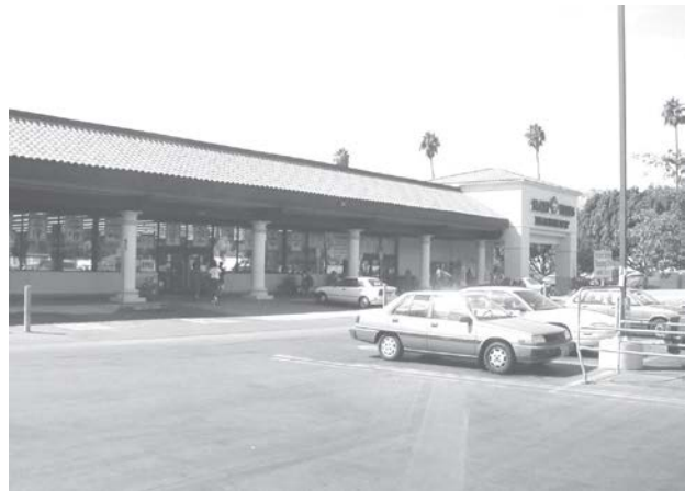
The Shopping Complex at Brockton and University Avenues
