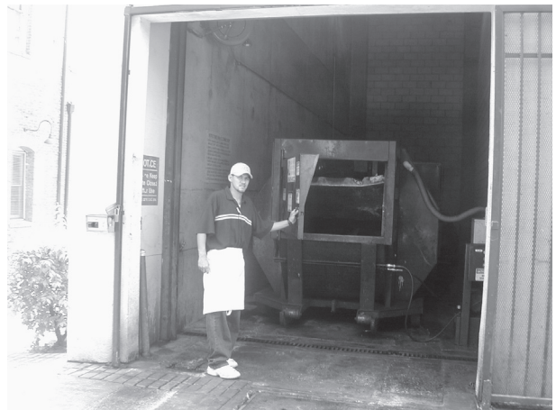
Alley walkways can also provide access to centralized trash compactors serving an entire block. These compactors are built into parking structures.
