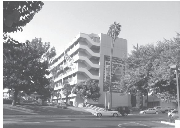
Riverside Community Hospital, 1960's wing
