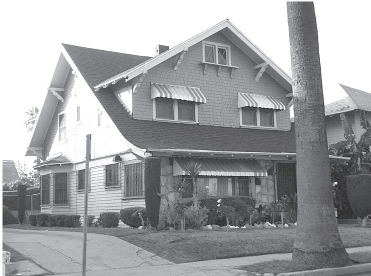
Inappropriate Porch Enclosure
