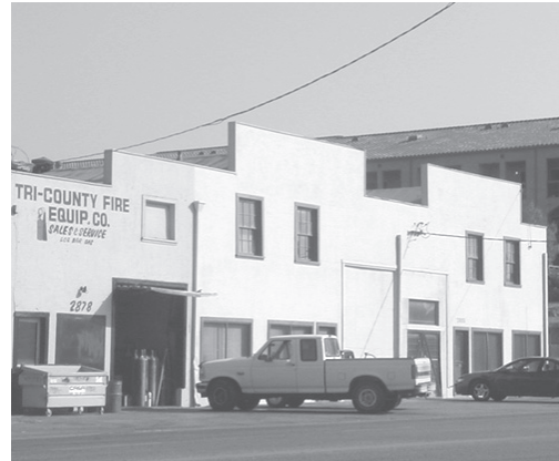
Tri-County Fire Equipment, 2878 N. Main Street
