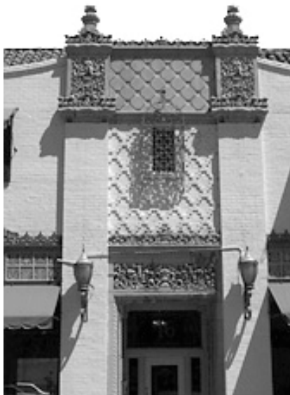
Examples of parapets and cornices
