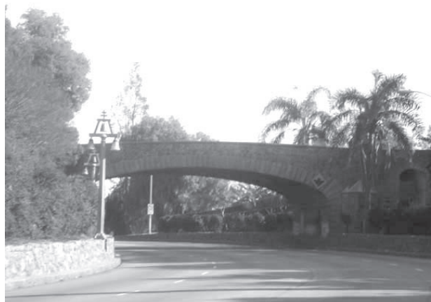
Mission Inn Avenue Historic Bridge
