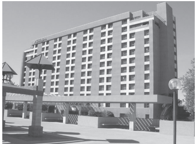
Existing Hotel at the Convention Center
