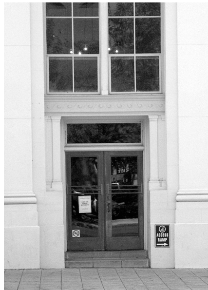
Clearly marked commercial entryway
