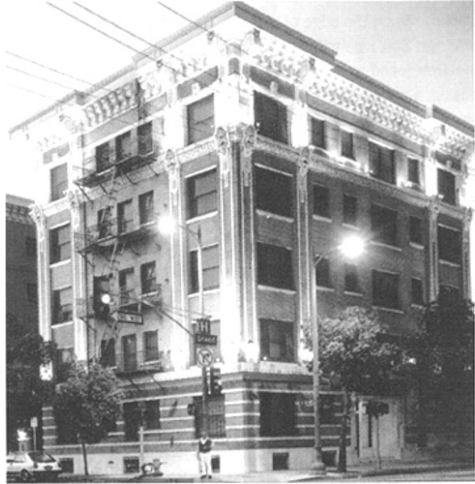
Example of lighting for historic buildings. Note the uplit cornice, the concealed lighting at the top of the pilasters and the decorative fixture at the street level.
