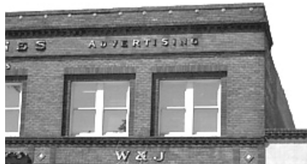
Examples of parapets and cornices
