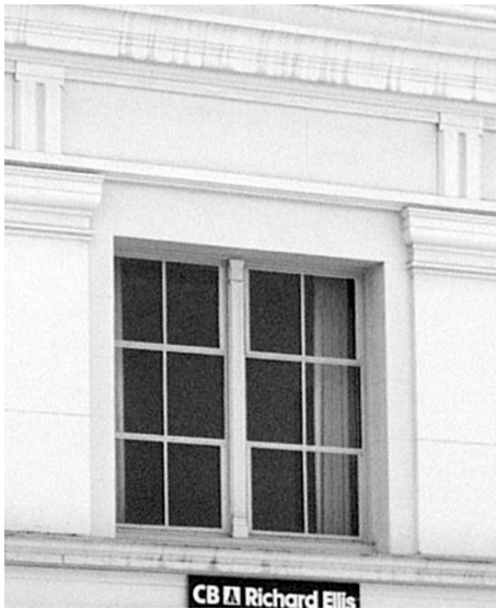
Divided light metal windows
