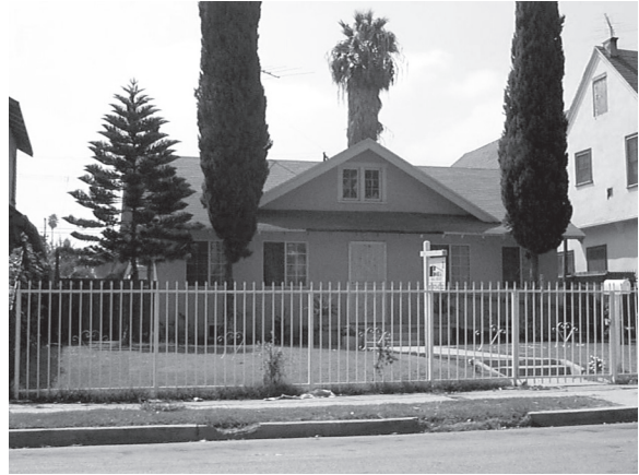
Inappropriate Metal Fencing
