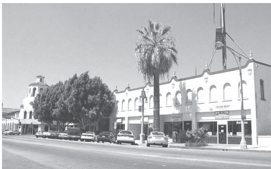
Stalder Building, Seventh Street Historic District.
