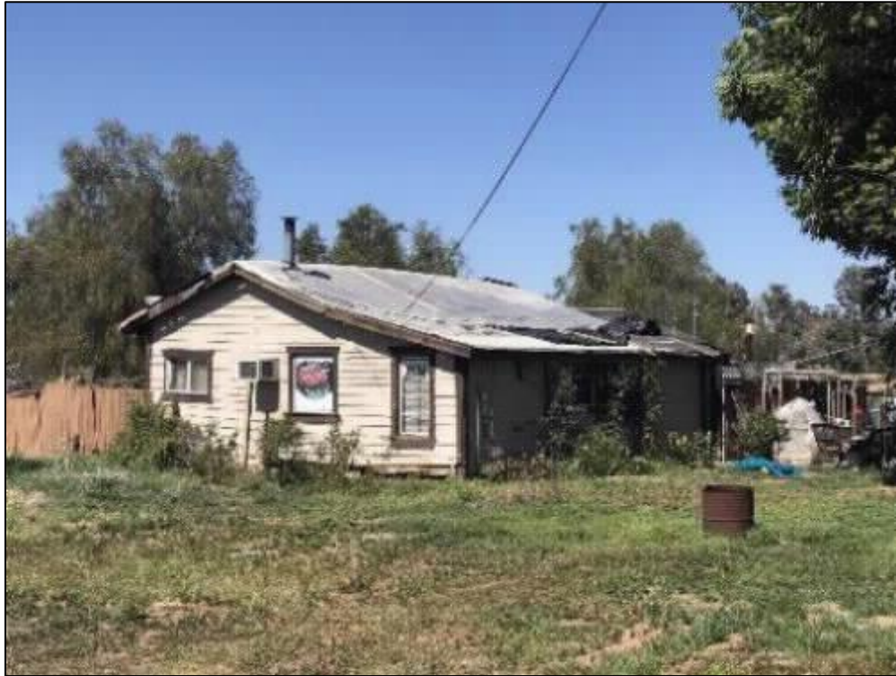
Figure 26. Overview of historic residential home, view northwest
