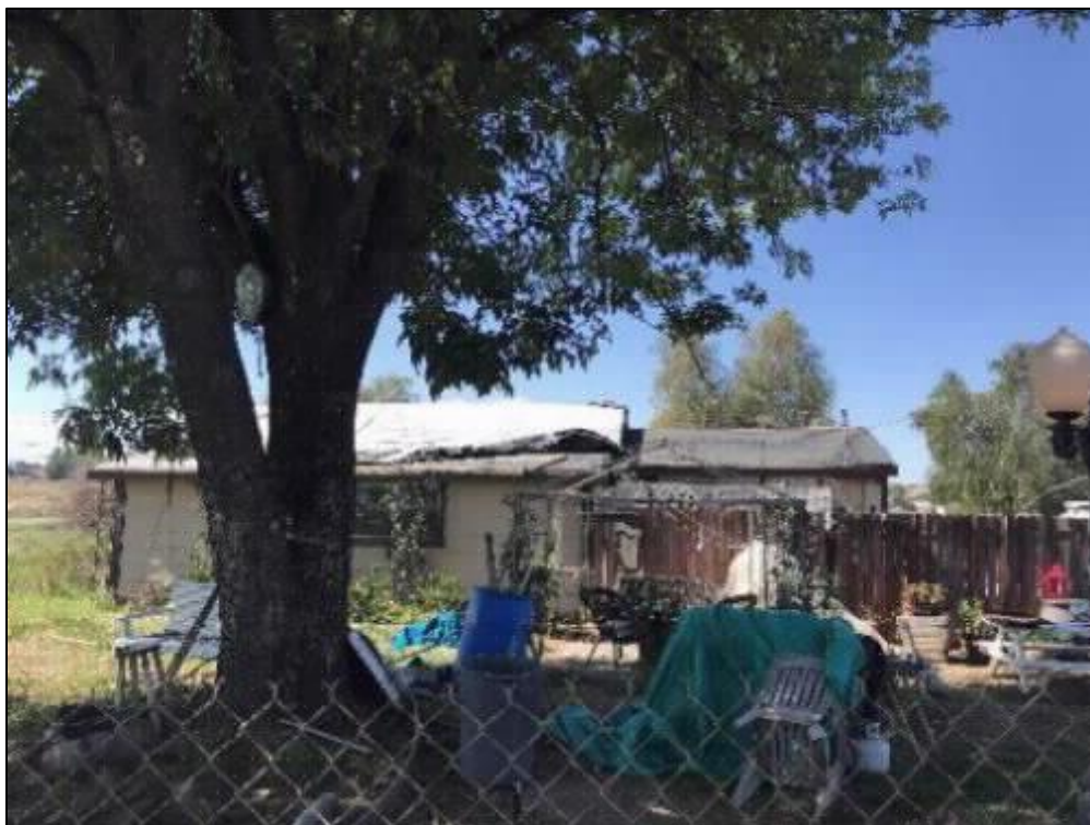
Figure 27. Overview of historic residence, view east
