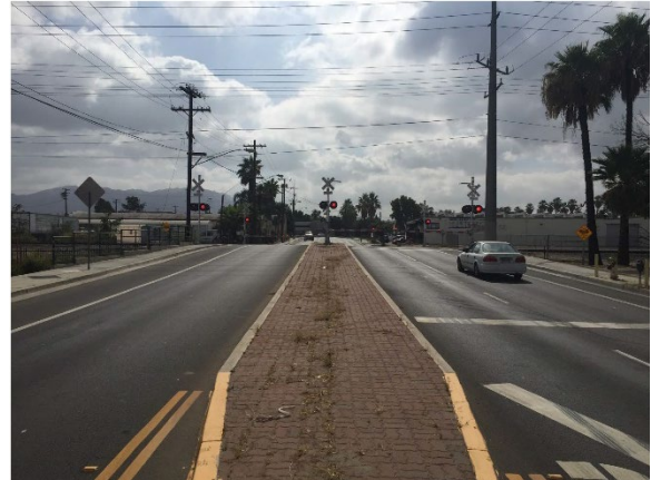
Figure 1: Existing Crossing with Gate Arms Down
