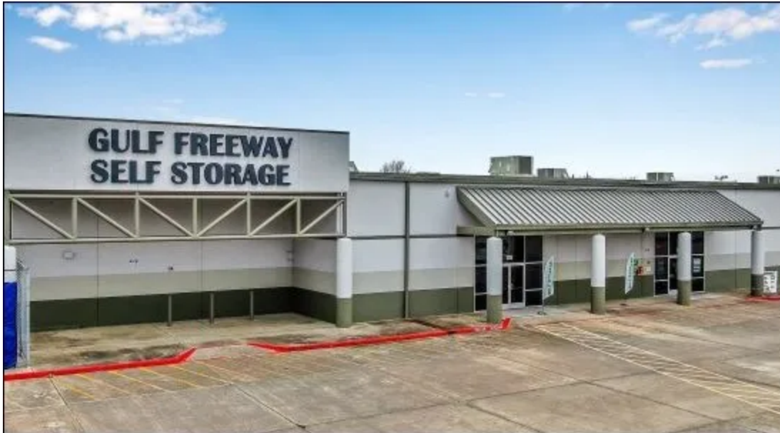
Gulf Freeway Self Storage in Houston
