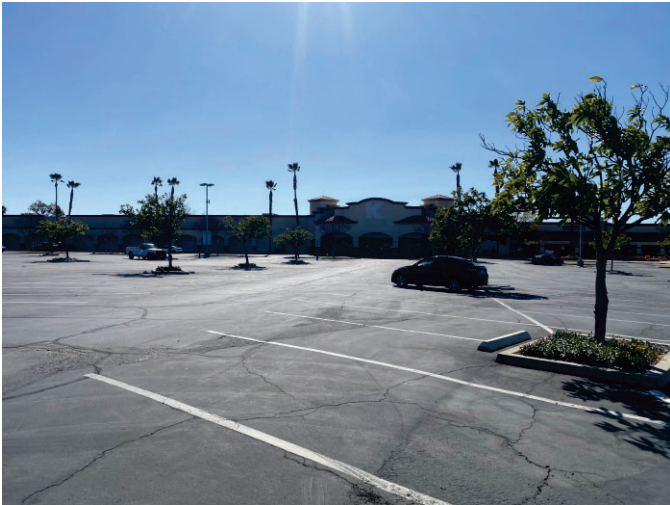
Photo 3: View from north side looking south.
