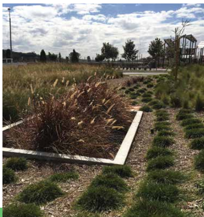
Open Top Planter - Filterra Bioscape
