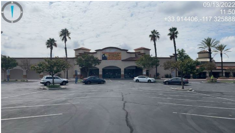
Photo 1: View South, showing current project site existing structures/buildings.
