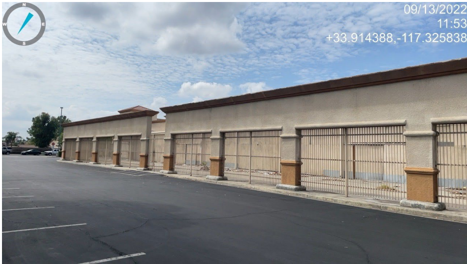
Photo 5: View Southwest of eastern side of project site existing structure.
