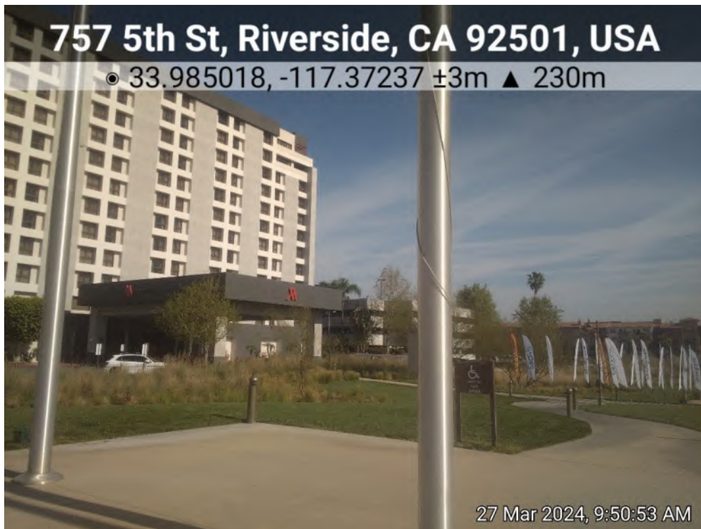
Photo 8. View of courtyard area and Marriot hotel parking area on the project site, facing northwest.
