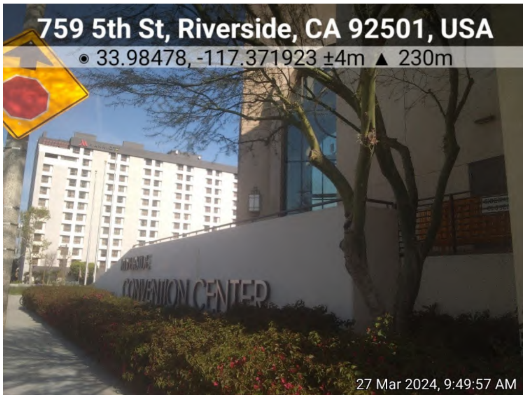
Photo 6. View of Convention Center entrance from 5 th Street along southwestern border, facing northwest.
