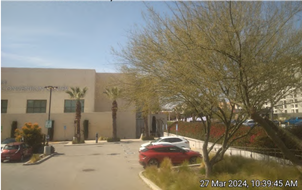
Photo 14. View of employees parking lot on the project site, facing southwest.
