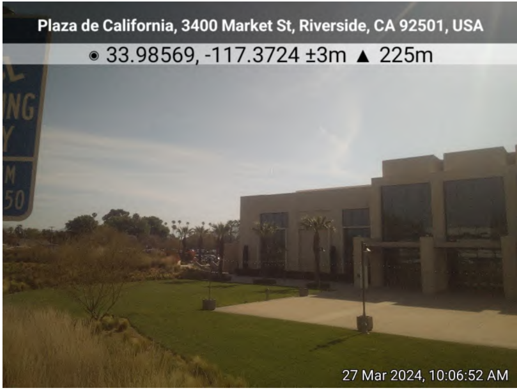
Photo 10. View of courtyard area on the project site, facing northeast.
