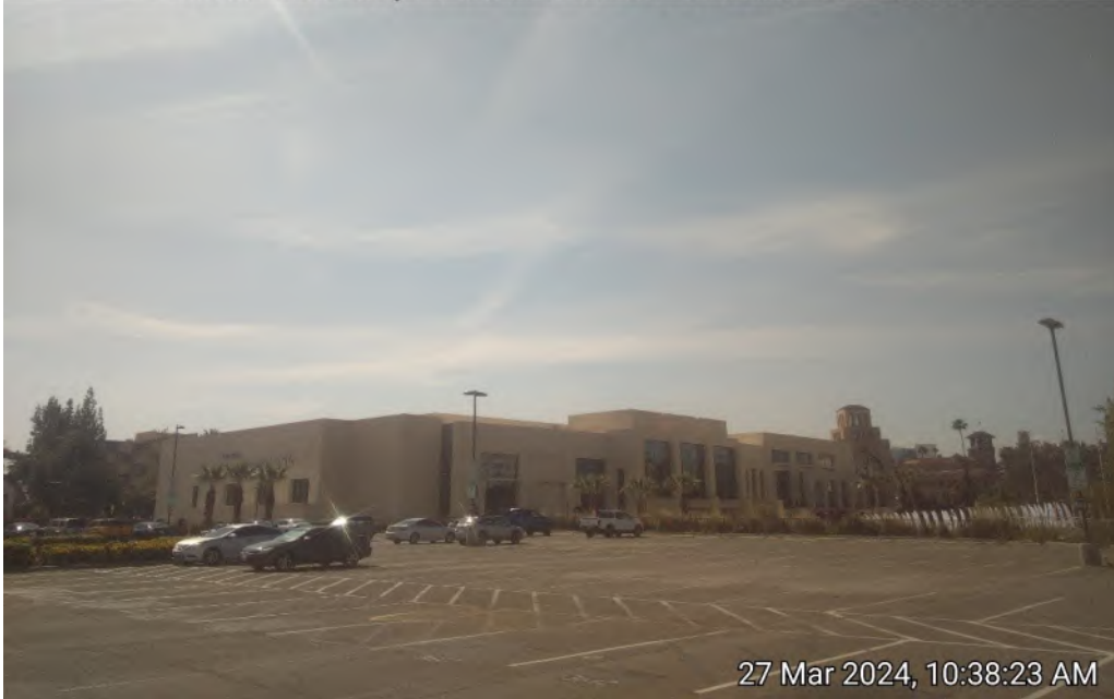
Photo 13. View of parking lot on the project site, facing southeast.
