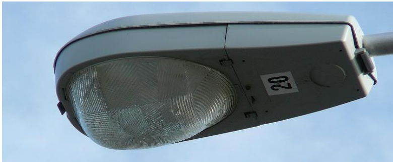
Old High Pressure Sodium Fixture (HPS)
