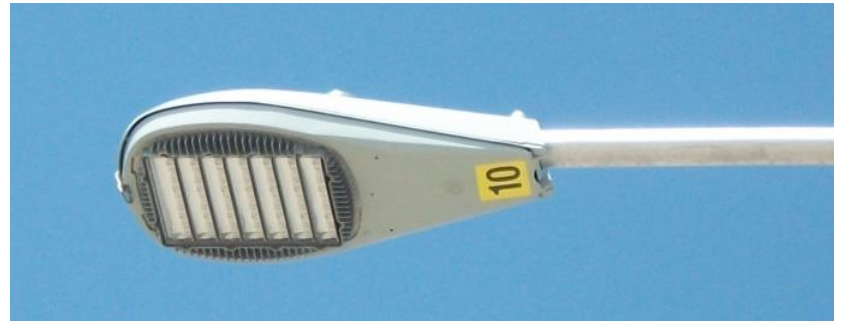
New Light Emitting Diode Fixture (LED)
